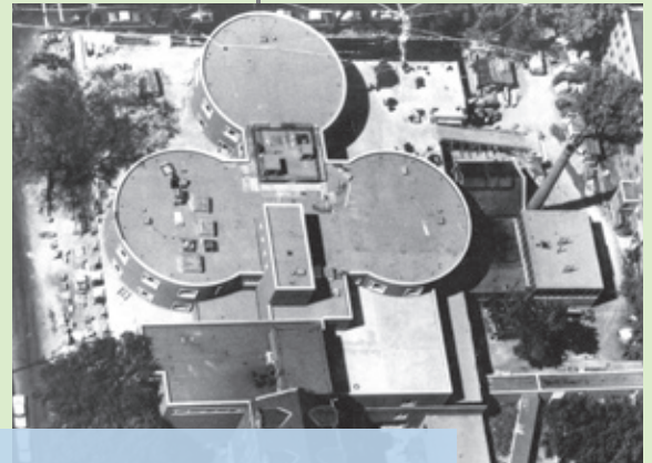
Modern Hospital magazine honors St. Luke's for the design of its innovative and function cloverleaf addition, locating the nurses station in the center with patient rooms it periphery.
