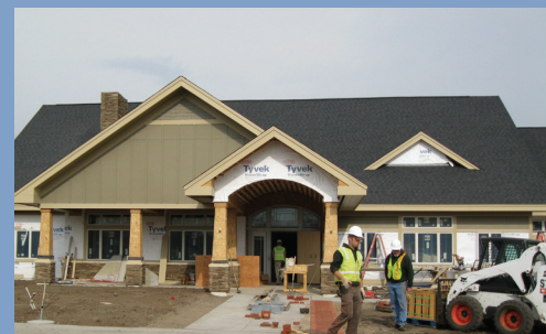
Construction of the Wedum Hospice will be complete in February 2012.
